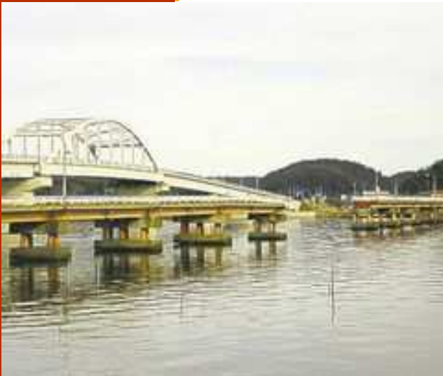
Hokota bridge: the old and the newly re-built one (in background)
